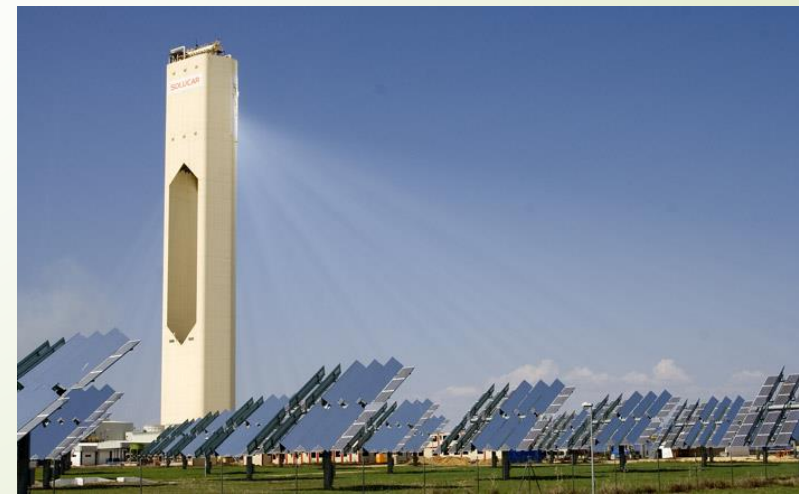
PS10 solar power tower - 11 megawatt, 624 large movable mirrors – Andalusia, Spain
